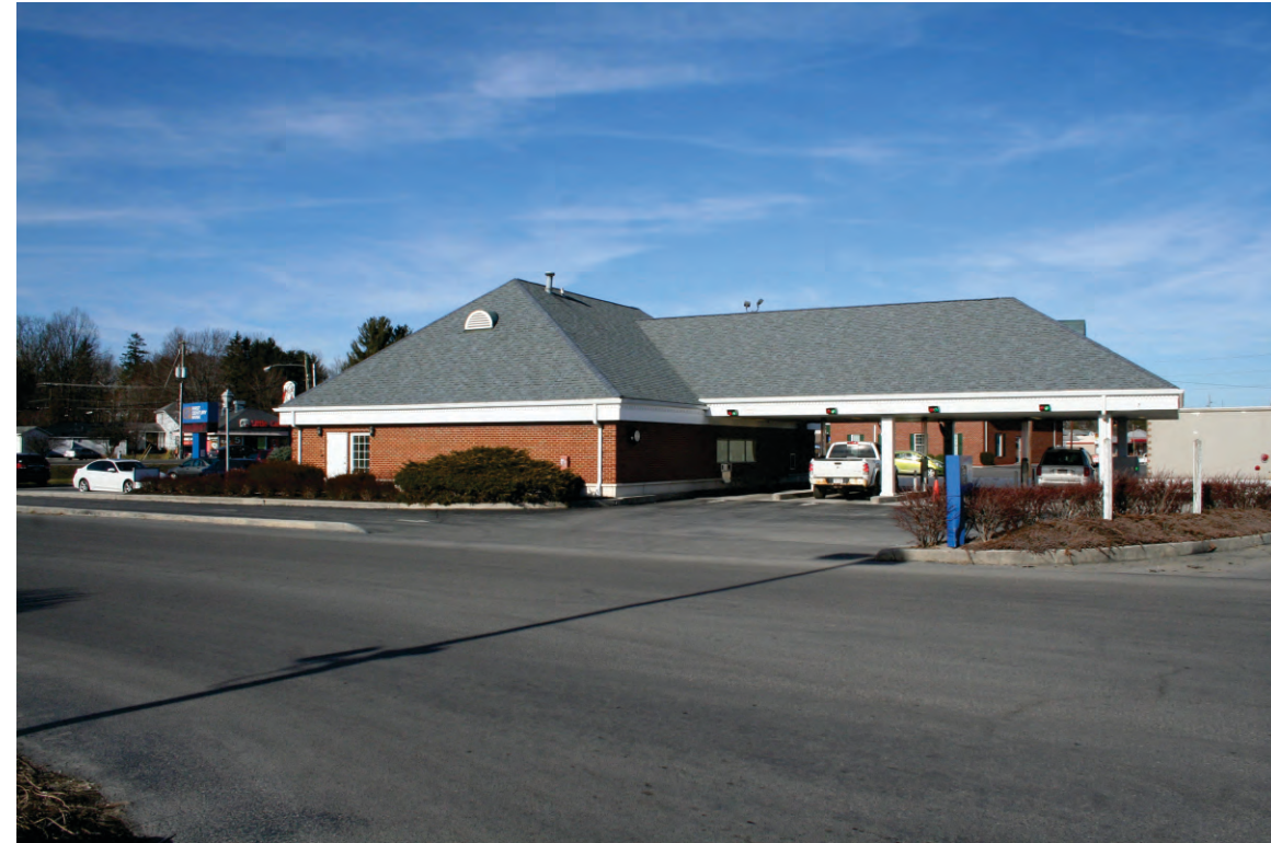
GENERAL NOTE: THIS PHOTO WAS TAKEN FROM THE NORTHEAST QUADRANT OF THE LOT
