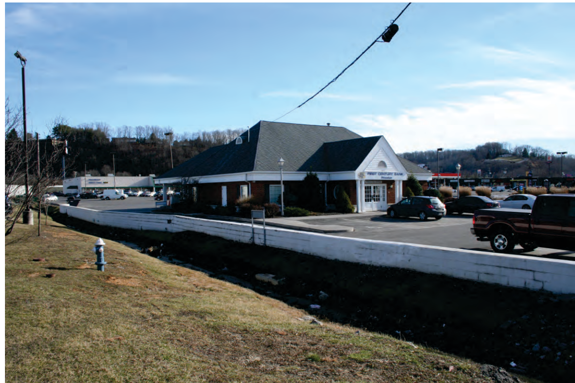
GENERAL NOTE: THIS PHOTO WAS TAKEN FROM THE SOUTHWEST QUADRANT OF THE LOT
